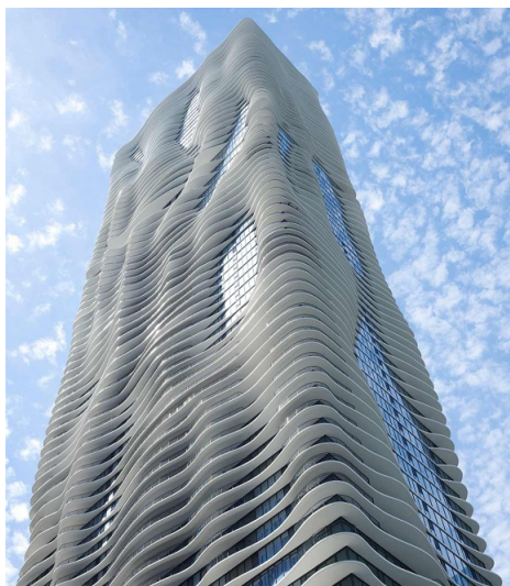
Figure 18: Aqua tower in Chicago, Illinois. Credits to Steve Hall © Hedrich Blessing
